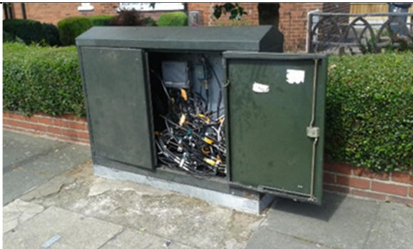
Exposed Wiring
