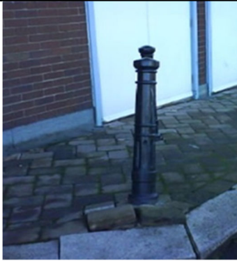
Damaged Bollard and Displaced Block Paving
