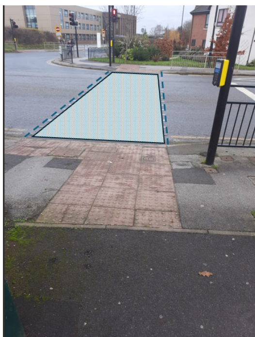
Signal crossing with tactile paving
