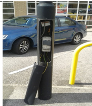
Exposed Wiring
