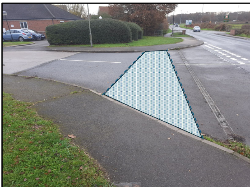
Dropped kerb at junction crossing point
