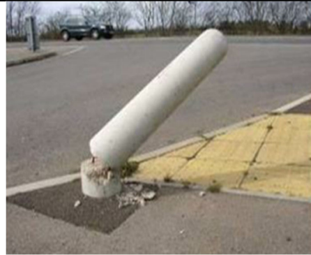
Damaged Bollard (overhanging Tactile Paved Crossing)
