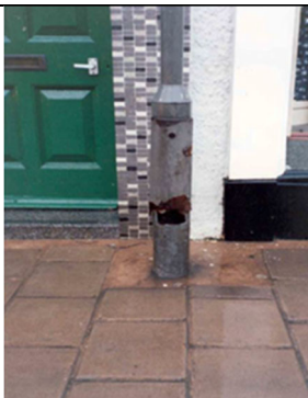
Corroded Column
