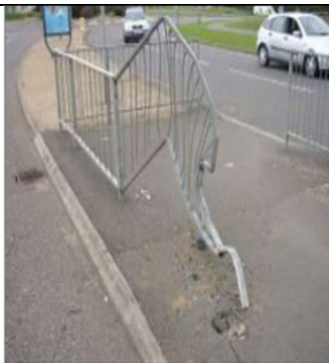
Damaged Pedestrian Barrier (at ped crossing location)
