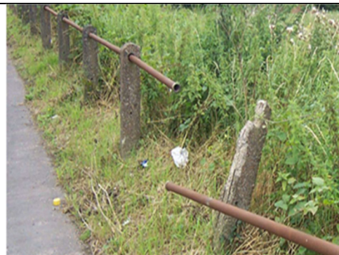
Damaged Fence (pole projecting into the highway)
