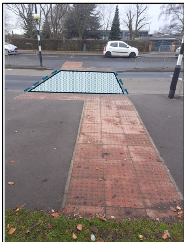
Beacon crossing with tactile paving
